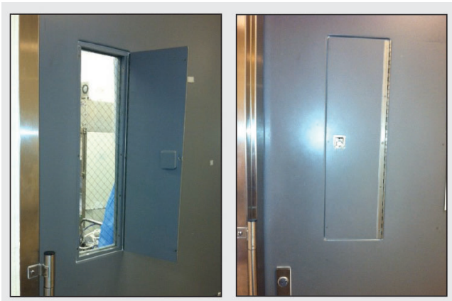
Figure 4.2.3.8 ARF Door Vision Panels and Hardware
