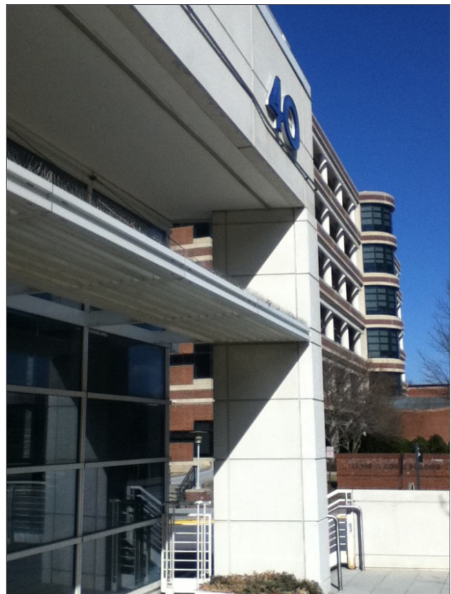
Figure 4.1.6 Sunshading at Building Entrance
