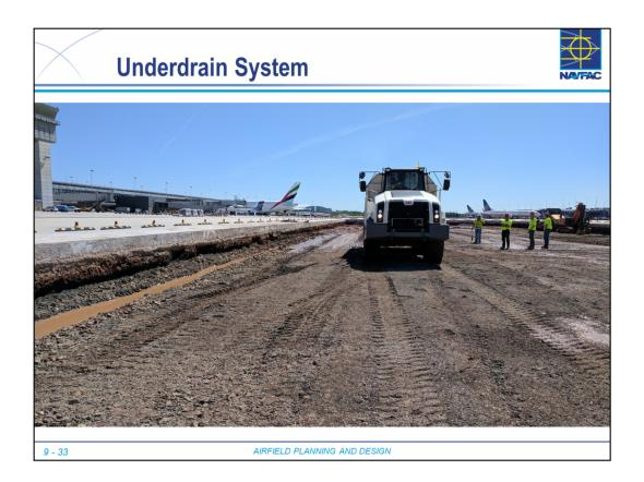
• Cut UD trench early to facilitate subgrade drainage
