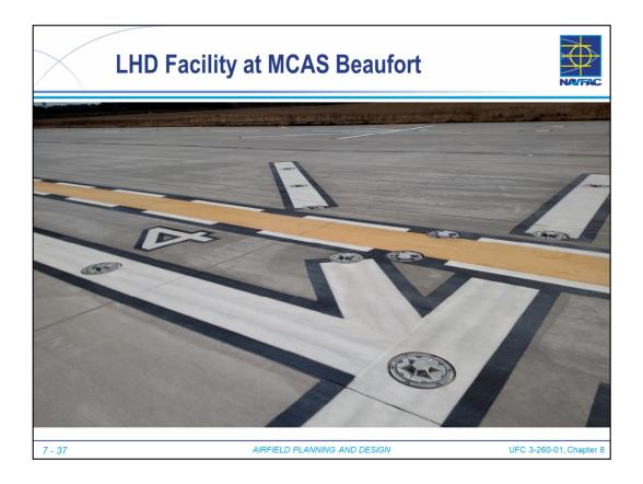
• Landing Spot 4 Marking and Lights with Tram Line through spot
