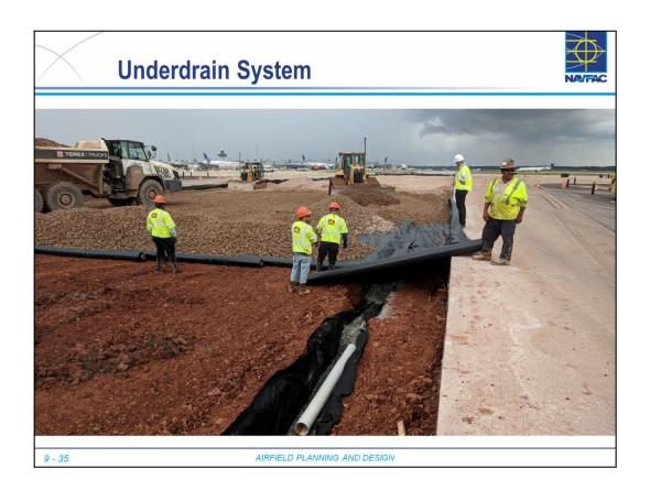
• Fabric in trench prior to pipe placement
