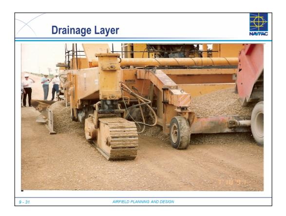
• Paver & spreader box used to distribute drainage layer material and reduce segregation
