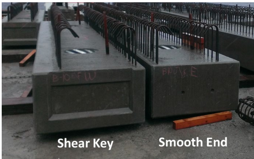
Precast Pile Cap Showing End Configurations
