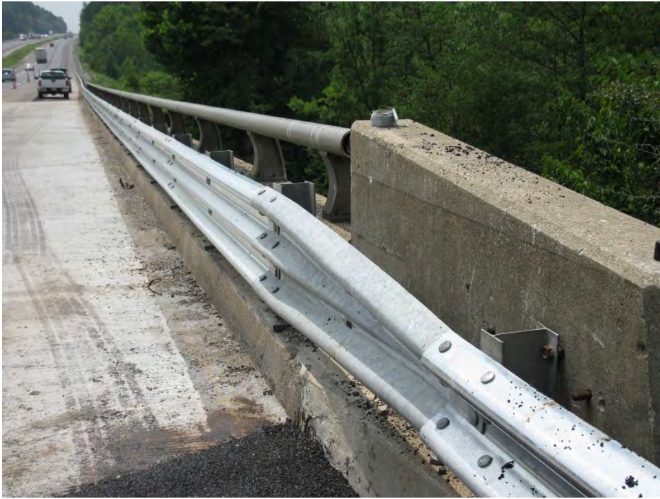
Figure 3.2-Bridge rail retrofit with thrie beam
