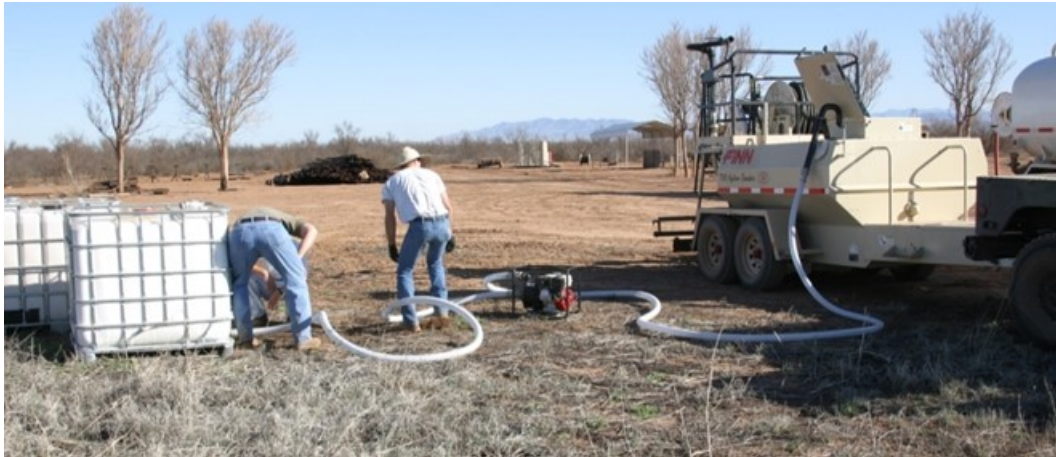
Figure 5-5 Filling Hydroseeder from Material Tote
