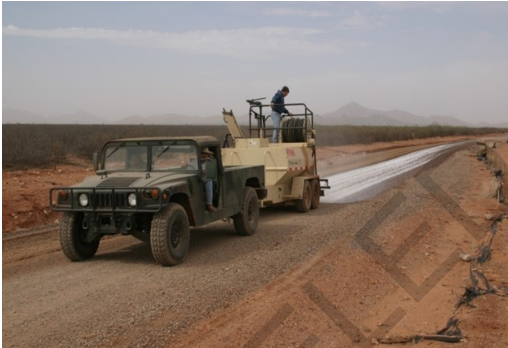
Figure 5-4 Applying Final Spray to Seal Road Surface After Compaction
