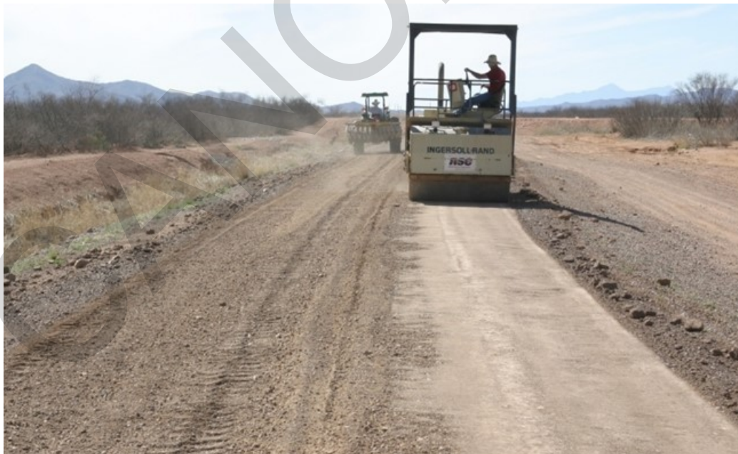
Figure 5-3 Compacting Road Surface After Mixing
