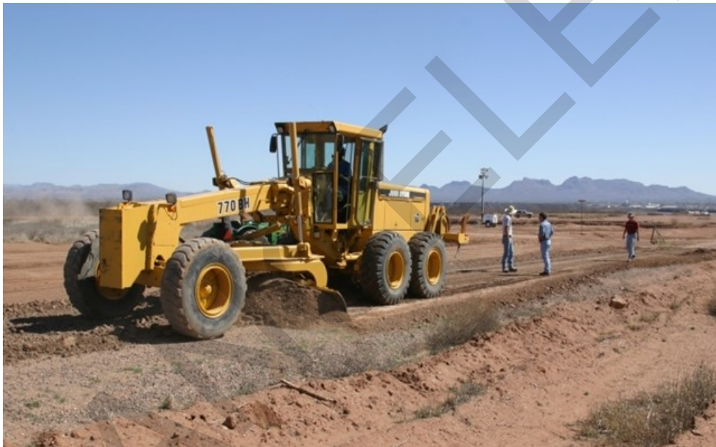
Figure 5-1 Grading Road Surface Prior to Treatment
