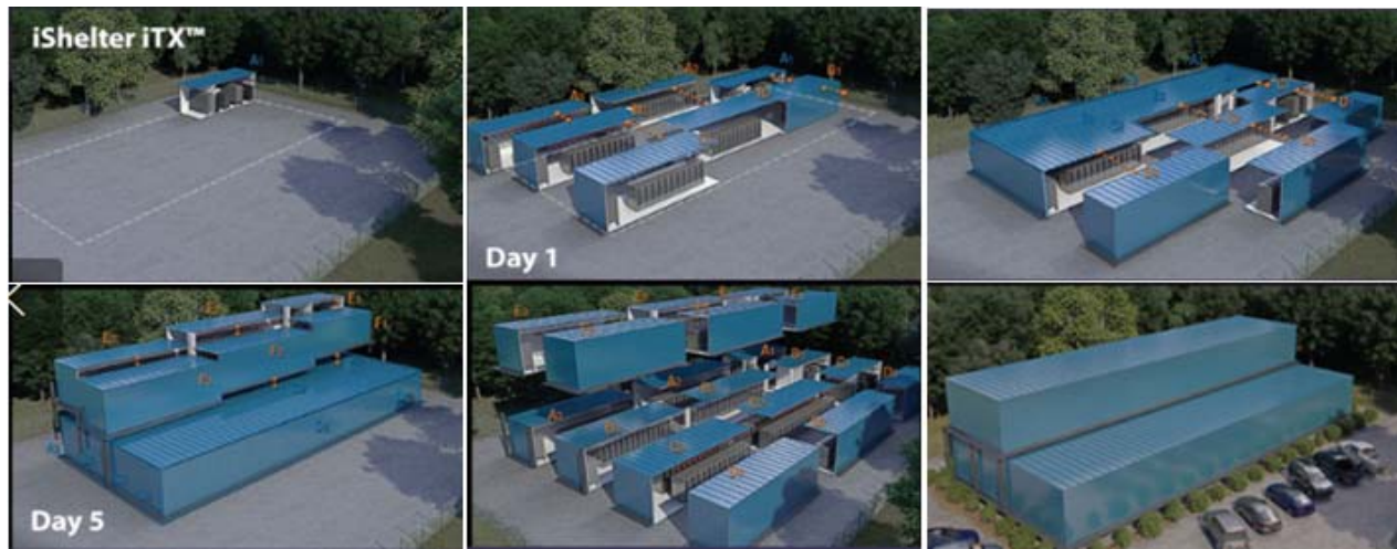
Figure 2 – pre-engineered Modular Data Center may be shipped assembled modules or “kit-of-parts” components
