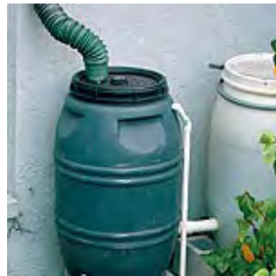
Figure A-11. Rain barrel used for simple irrigation.
