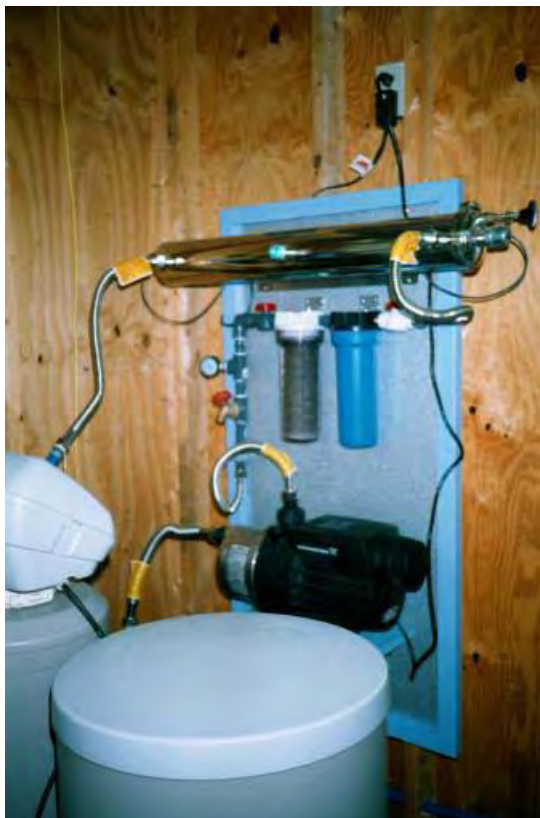
Figure A14. Typical treatment installation of an on-demand pump, 5-micron fiber filter, 3-micron activated charcoal filter, and an ultraviolet lamp (top) (source: TWDB 2005).
