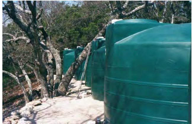
Figure A8. Low-profile 5,000-gal polypropylene tanks (source: TWDB 2005).
