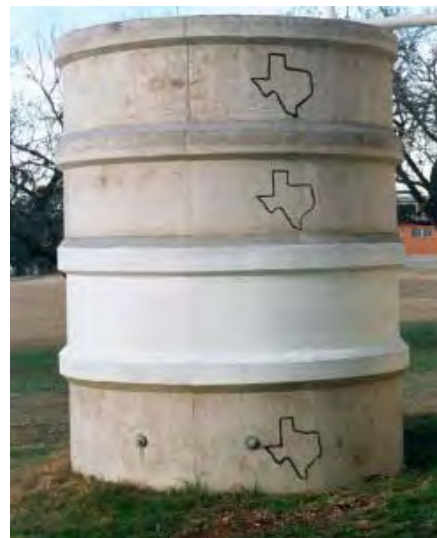
Figure A10. Concrete tank fabricated by stacking rings of concrete (source: TWDB 2005).
