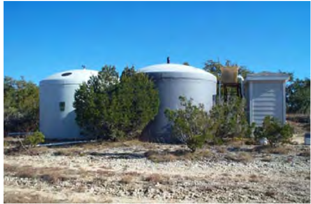
Figure A7. Two 10,000-gal fiberglass tanks (source: TWDB 2005).
