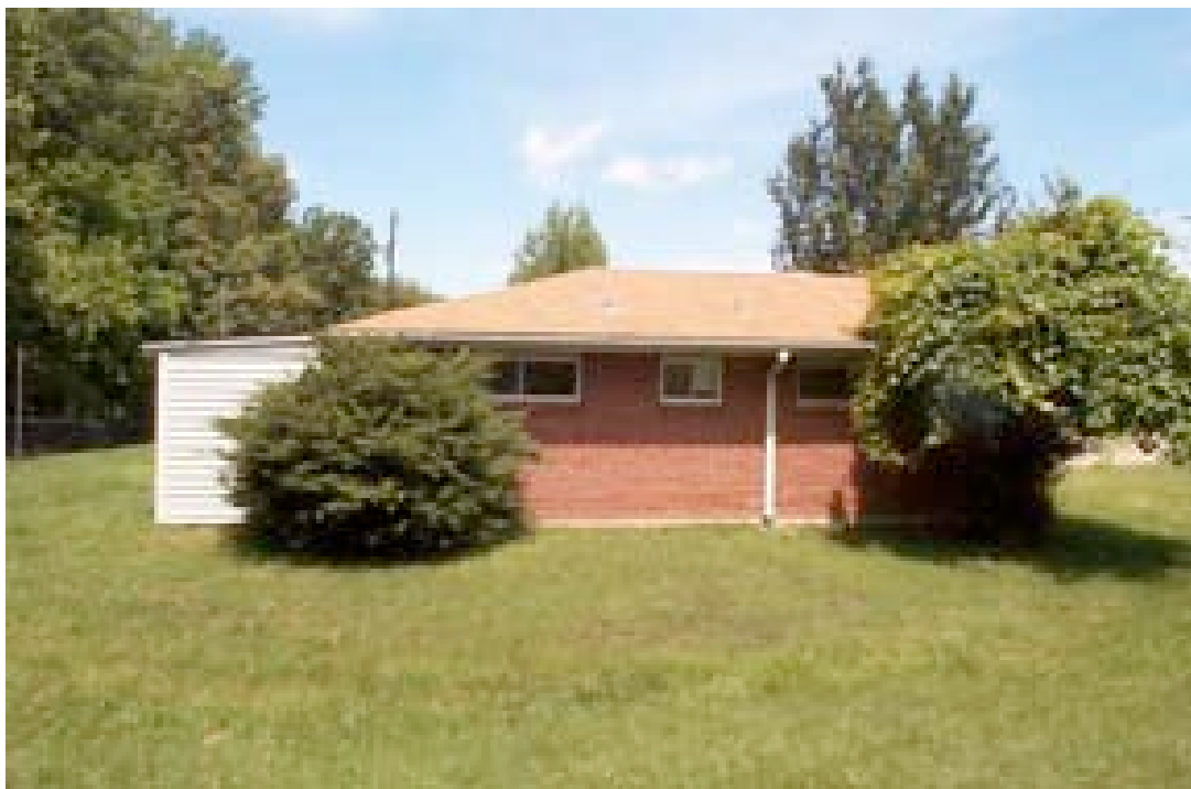
Figure 3-3. Side view of FHU duplex at Fort Campbell.
