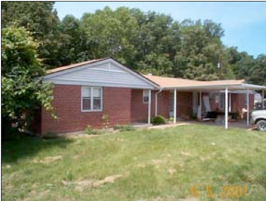
Figure 3-1. Front of FHU duplex at Fort Campbell.
