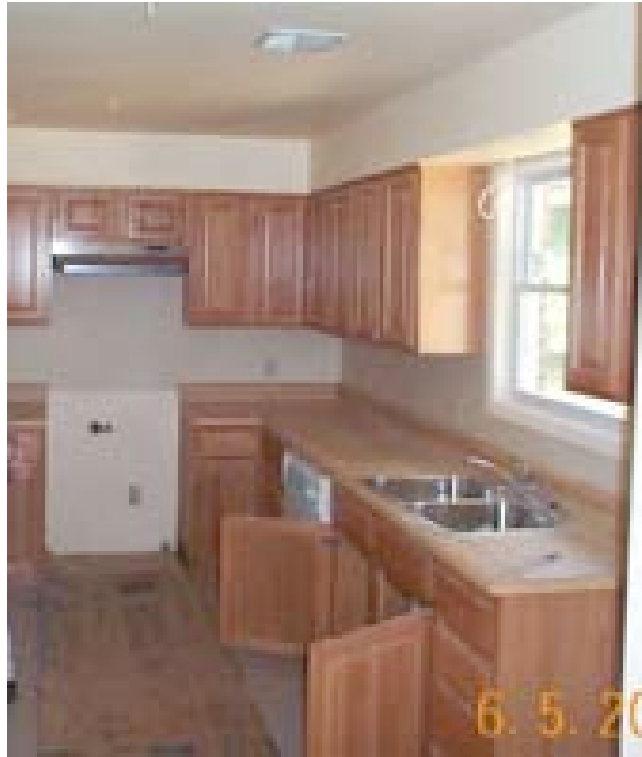
Figure 3-12. Remodeled kitchen in Fort Campbell duplex.
