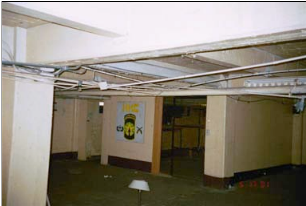
Figure 2-9. Basement of selected building at Fort Bragg.
