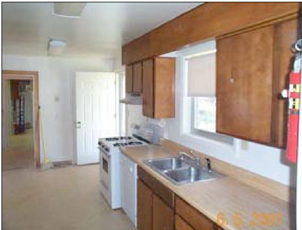
Figure 3-5. Kitchen in FHU duplex at Fort Campbell.
