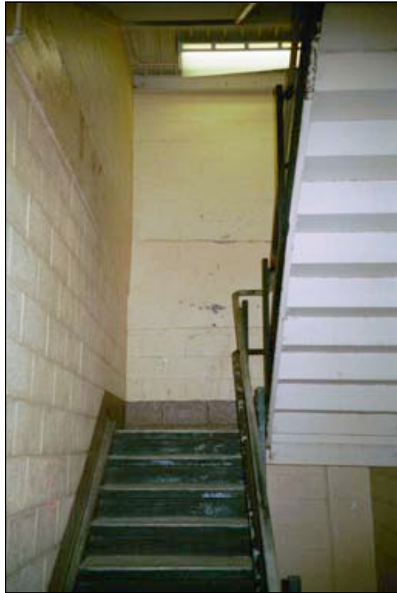
Figure 2-6. Stairs inside selected building at Fort Bragg.
