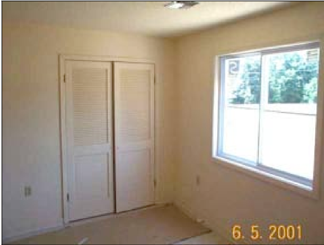
Figure 3-14. Remodeled bedroom in Fort Campbell duplex.
