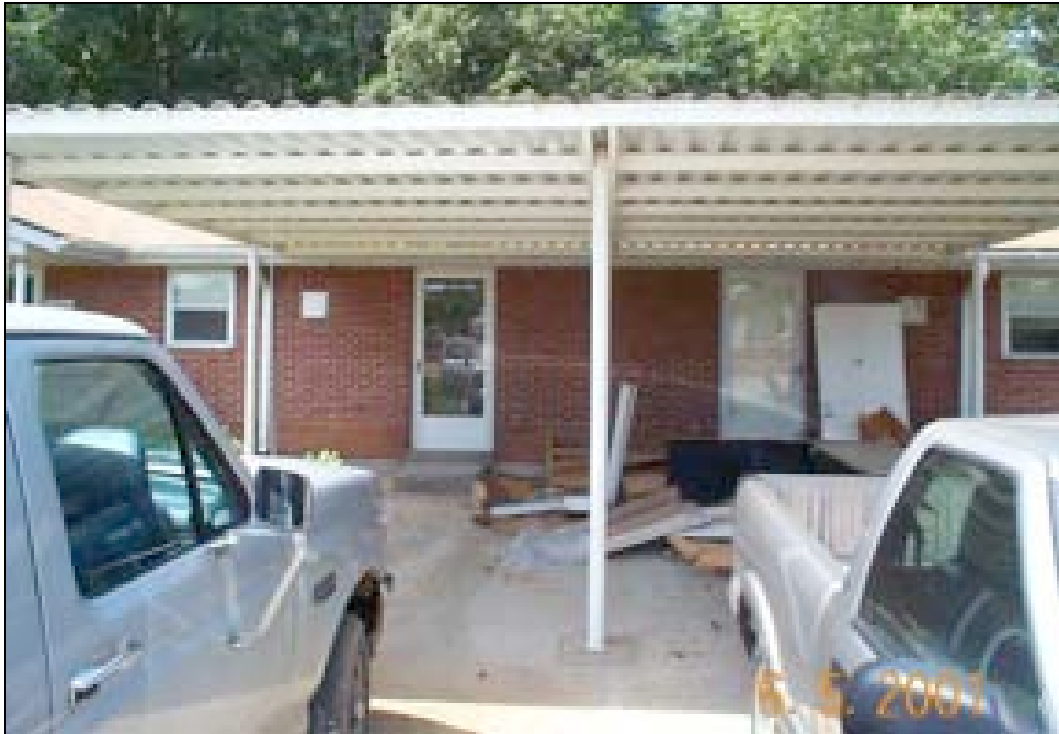
Figure 3-2. Carport of FHU duplex at Fort Campbell.
