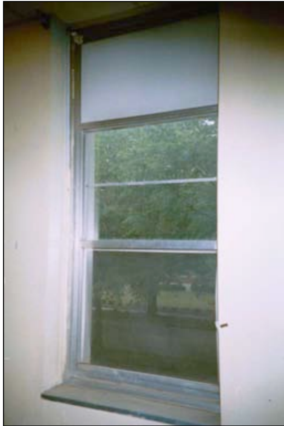
Figure 2-8. Window inside selected building.
