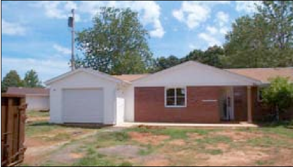
Figure 3-10. Front of remodeled FHU duplex at Fort Campbell.
