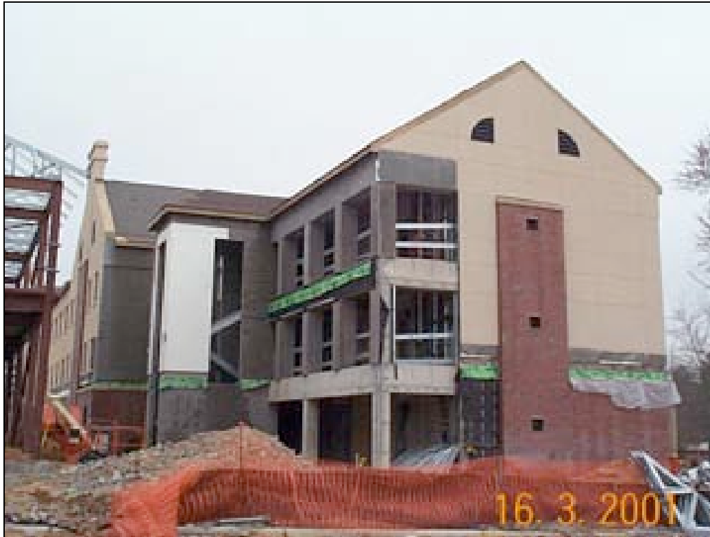
Figure 4-4. Barracks remodeling project at Fort Bragg.
