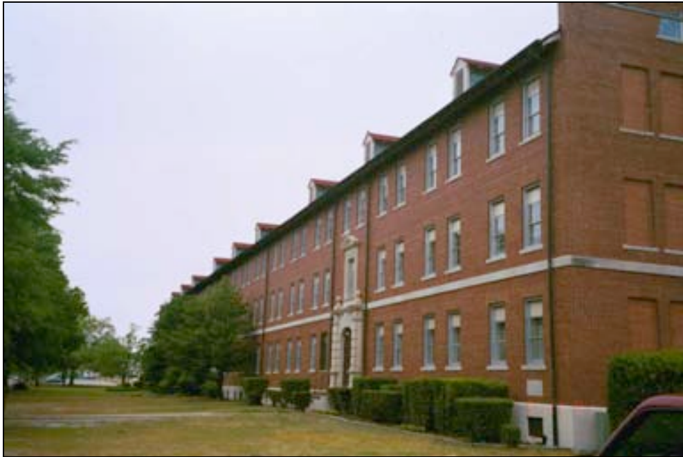
Figure 2-2. Front facade, selected building at Fort Bragg.
