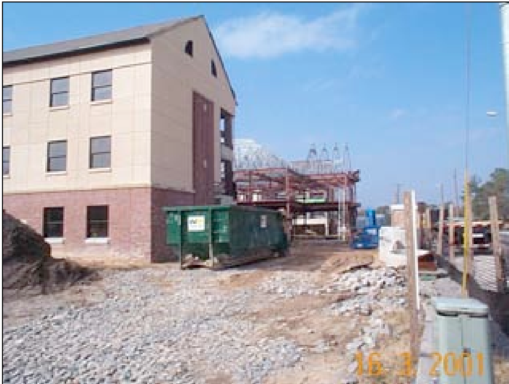
Figure 4-6. Another view of rolling-pin barracks remodeling.
