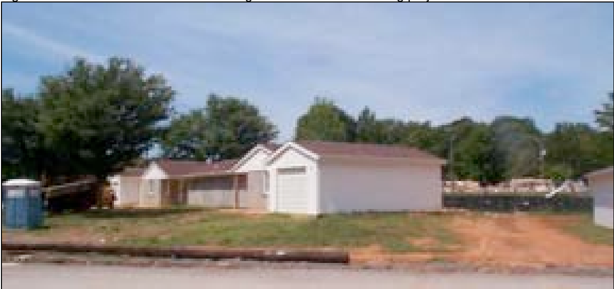
Figure 3-9. Remodeled FHU duplex at Fort Campbell.
