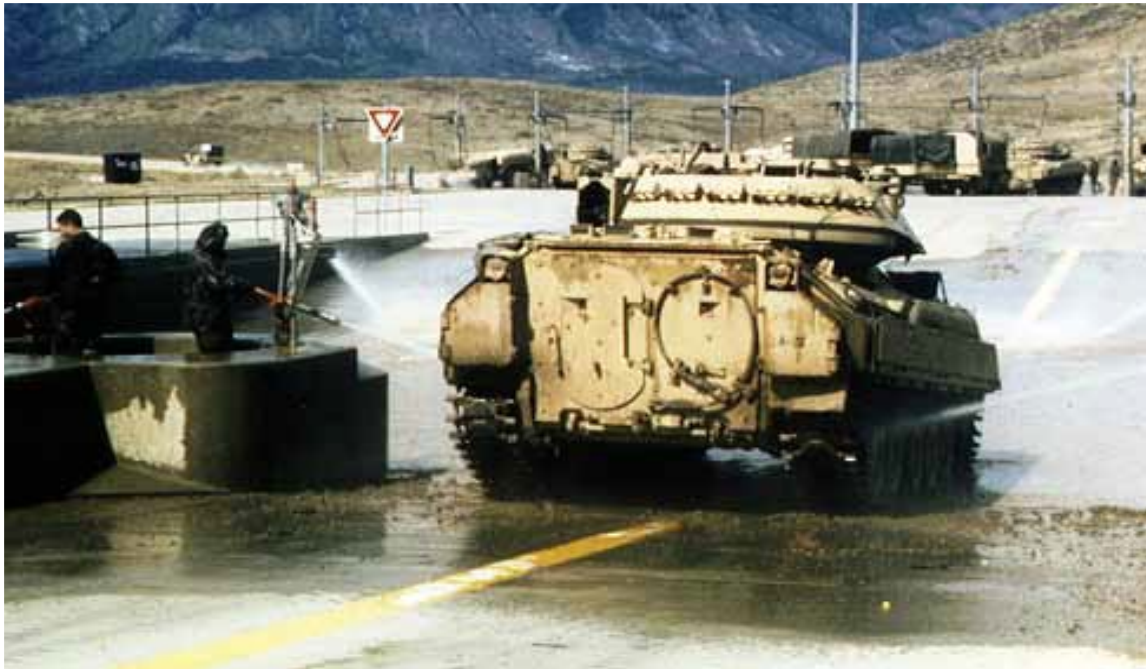
Figure A-1. A major user of recycled water are installation Central Vehicle Wash Facilities such as this one at Fort Carson, Colorado.
