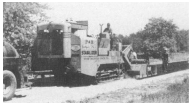
Figure 4-46. Multiple rotary mixer.
