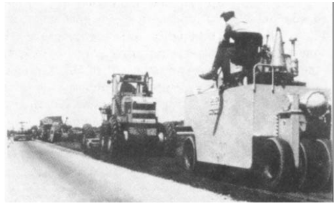
Figure 4-52. Spreading and compacting train.
