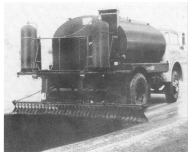
Figure 4-51. Distributor applying asphalt.
