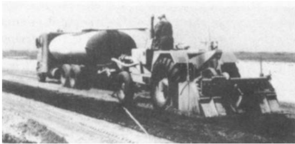
Figure 4-48. Single-shaft rotary mixer with asphalt supply tank.
