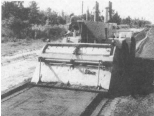
Figure 4-49. Single-shaft rotary mixer without asphalt.
