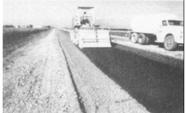
Figure 4-39. Rotary mixer on primary road project.
