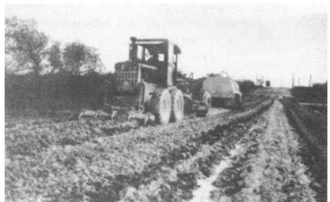
Figure 4-33. Grader-scarifier cutting slurry into stone base.
