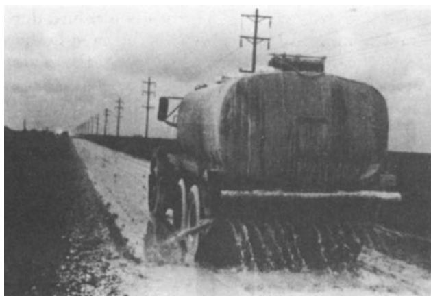
Figure 4-31. Spreading of lime slurry.
