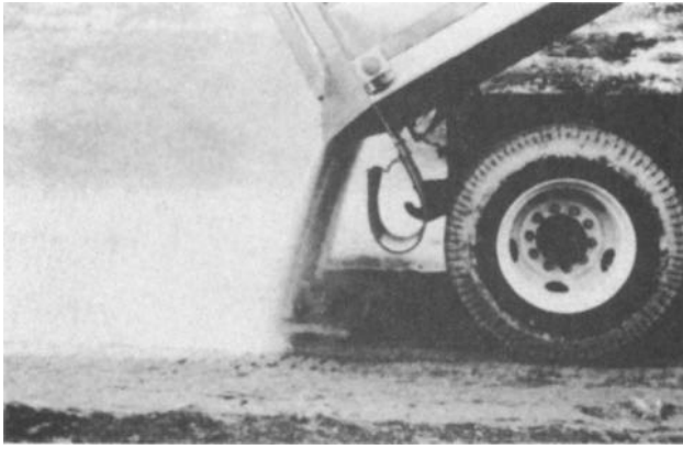
Figure 4-28. Spreading of granular quicklime.
