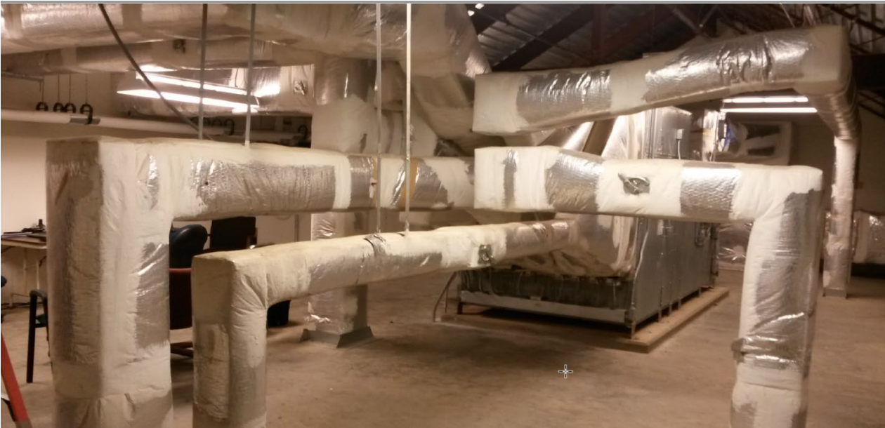
Multizone air handlers mix a zone specific air temperature for each zone, which has its own dedicated duct
