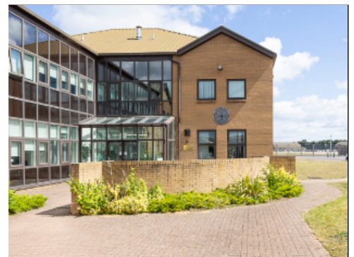
Pavers and Screen Wall
