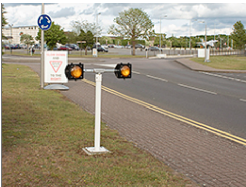
Signal at Special Intersection
