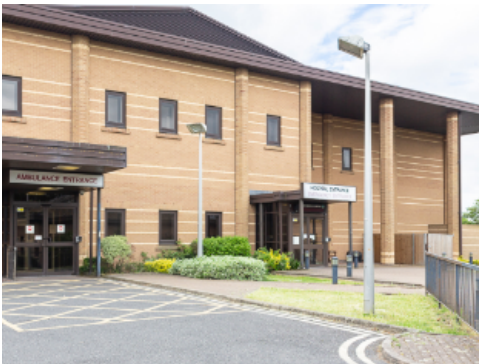
Lighting at Entry
