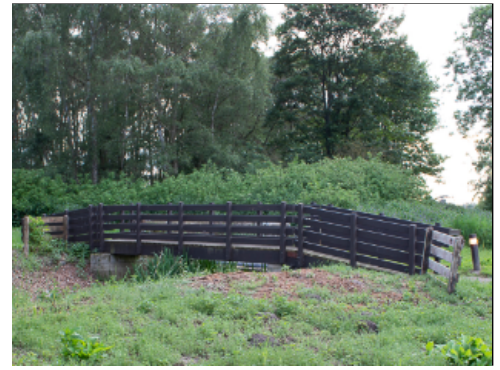
Ramp at Bridge
