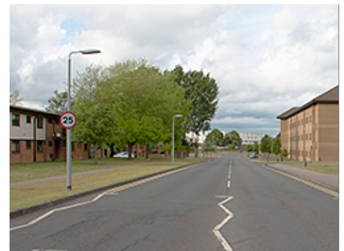
Detached Sidewalk with Landscaping
