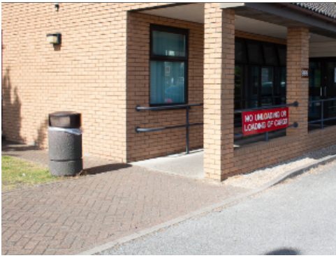
Ramp at Entry
