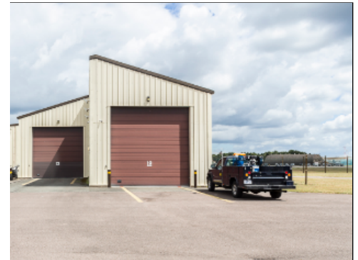
Parking Adjacent to Workspace
