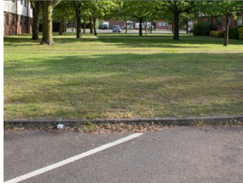
Concrete Curb at Grass
