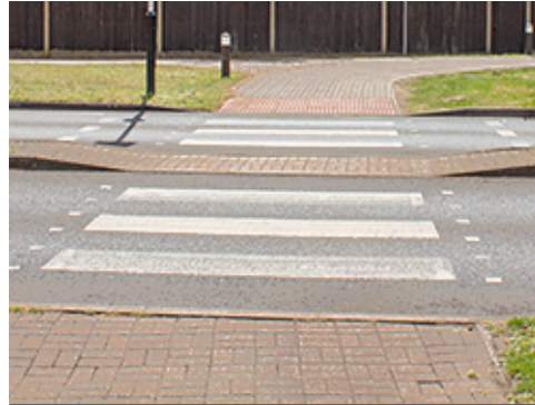
Curb Ramp at Crosswalk
