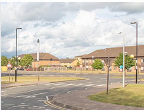
Buried Utility Lines
