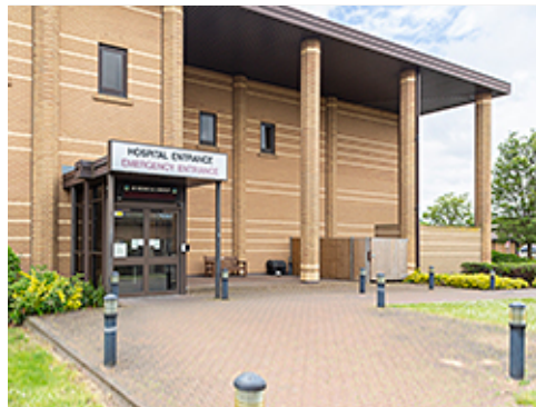
Plaza at Group 1 Entrance
