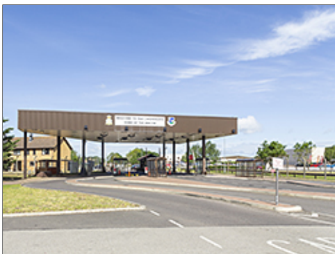
Arterial at Main Gate
