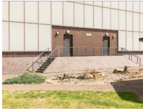
Stairs to Pavilion
