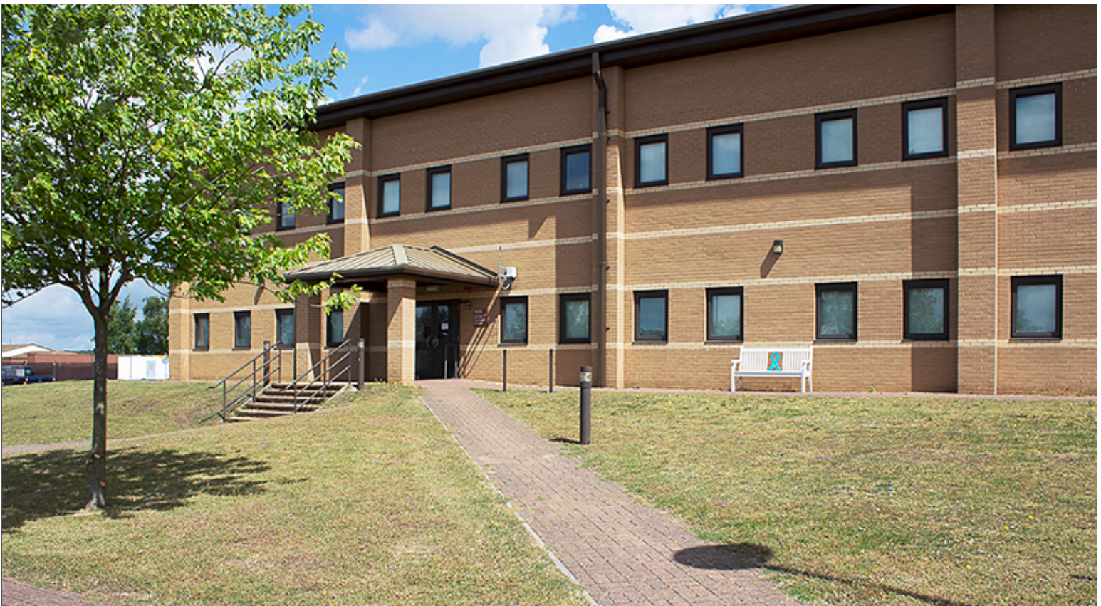
Ramp and Stair to Building
