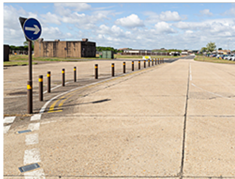
Concrete Paving at Group 3
