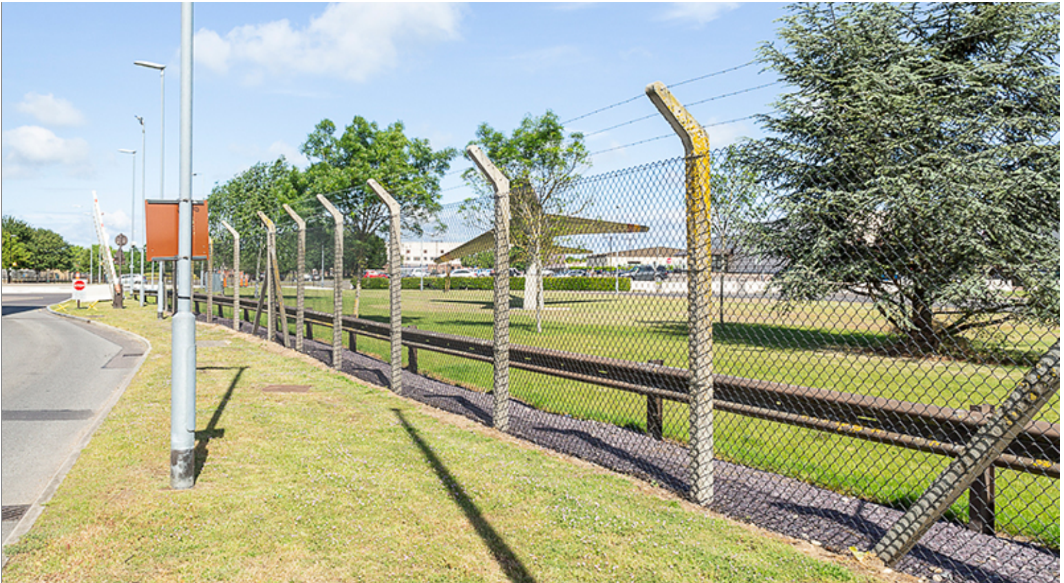
Perimeter Fence Adjacent to Main Gate
