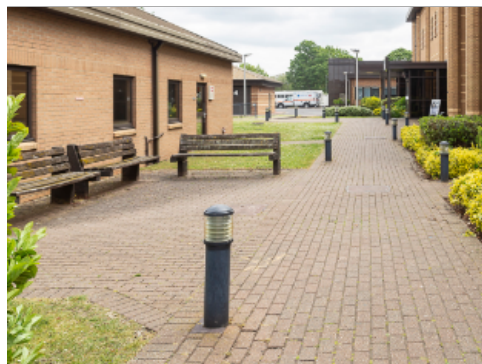
Pavers with Lighted Bollard
