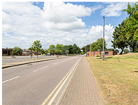
Sidewalk with Unit Pavers
