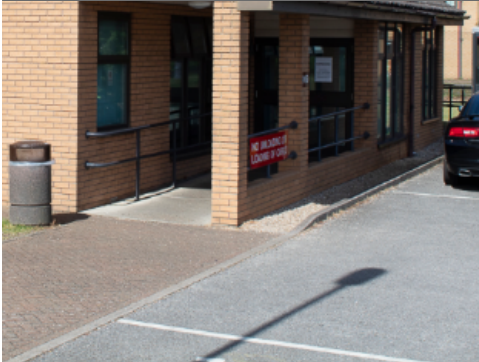
Lowered Curb for Access
