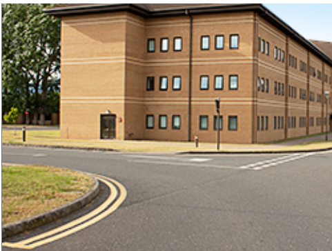
Striping at Curb
