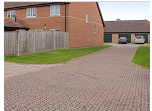
Decorative Interlocking Pavers at Group 4
