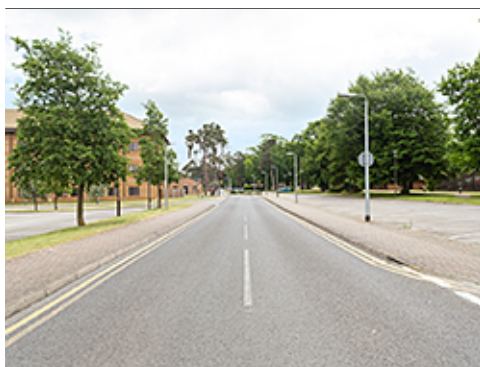
Group 2 Typical Frontage
