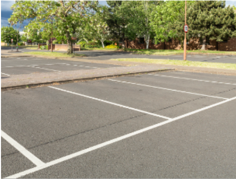
Painted Stripes on Pavement
