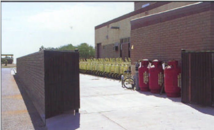
Provide an enclosure wall and gate to screen outdoor storage from public view
