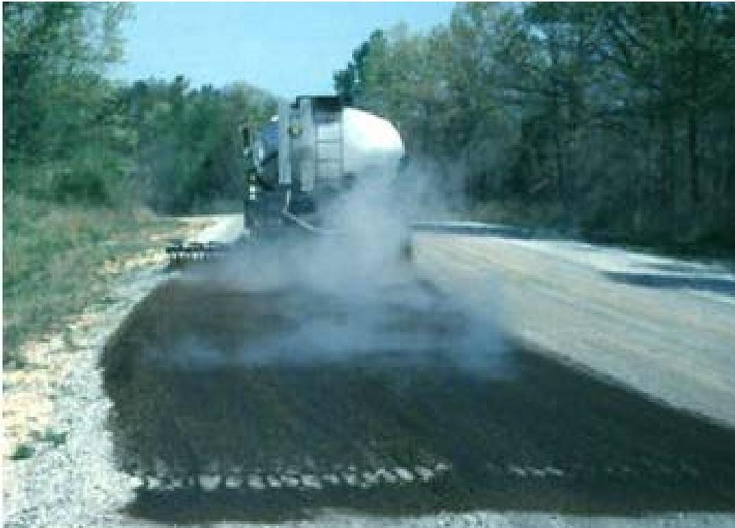
**Figure A-4. Various products can be applied for dust control. Here, soybean oil is being applied to a properly graded and very heavily trafficked main supply route at Fort Campbell, Kentucky.**
