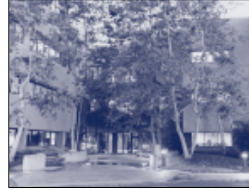
Photo courtesy of The City of San Diego's Ridgehaven Green Building Demonstration Project
