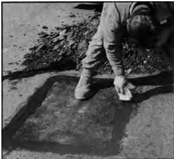
Figure 3.13. Sealing edges of the patch
