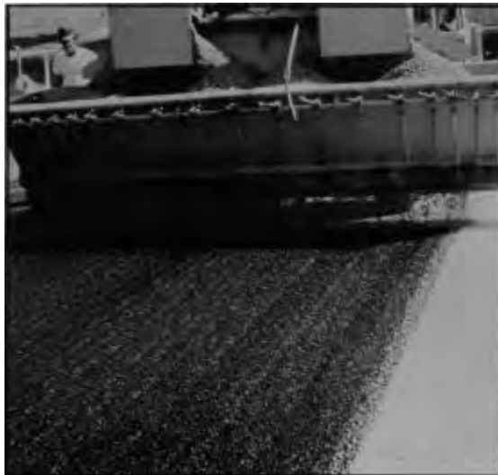
Figure 5.2. Applying aggregate with self-propelled hopper-type spreader
