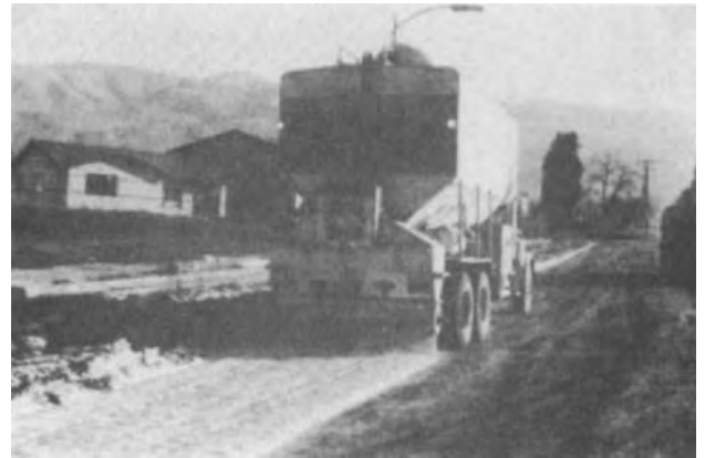
Figure 4-27. Distribution of quicklime from mechanical spreader on city street.
