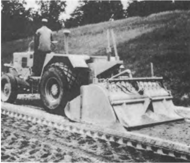
Figure 4-1. Transverse single-shaft mixer processing soil-cement in place. Multiple passes are required.
