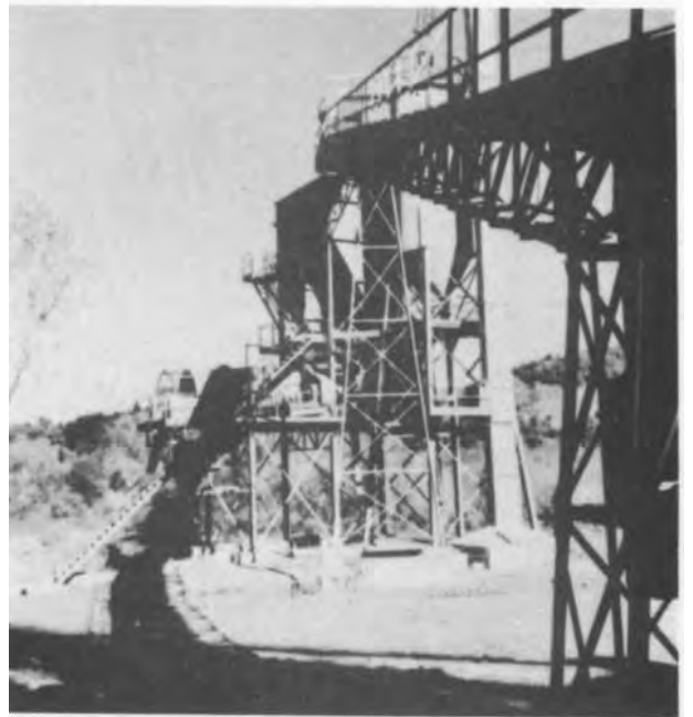
Figure 4-5. Batch-type central plant used for mixing soil-cement.
