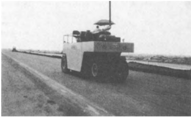
Figure 4-42. Pneumatic roller completes compaction of LCF base.
