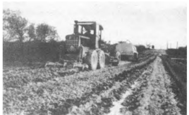
Figure 4-33. Grader-scarifier cutting slurry into stone base.
