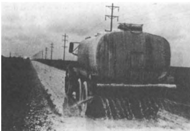
Figure 4-31. Spreading of lime slurry.
