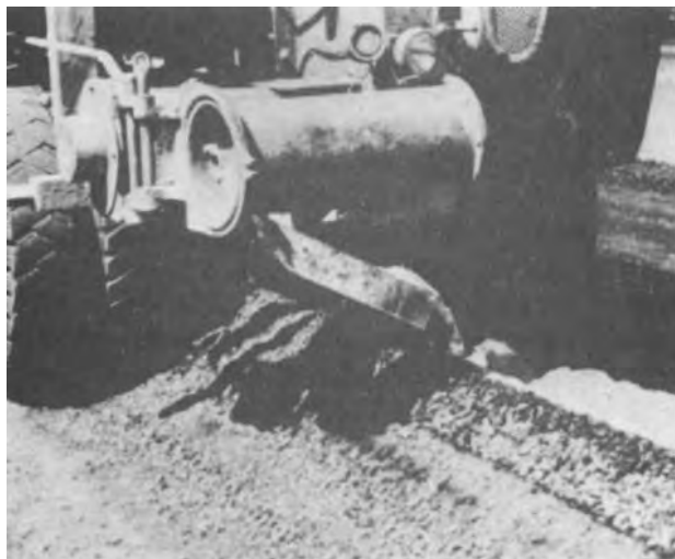
Figure 4-9. Windrow-type mechanical spreader placing cement on windrow.
