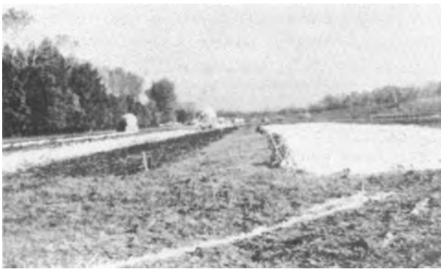
Figure 4-16. Off-site mixing pads for Mississippi River levee repair project.
