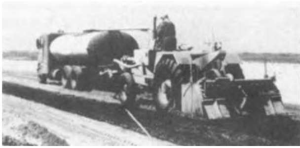
Figure 4-48. Single-shaft rotary mixer with asphalt supply tank.
