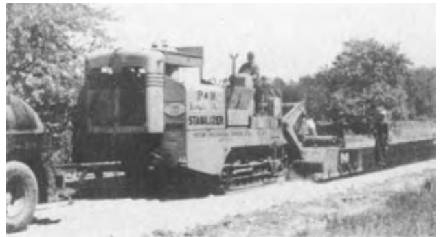
Figure 4-46. Multiple rotary mixer.
