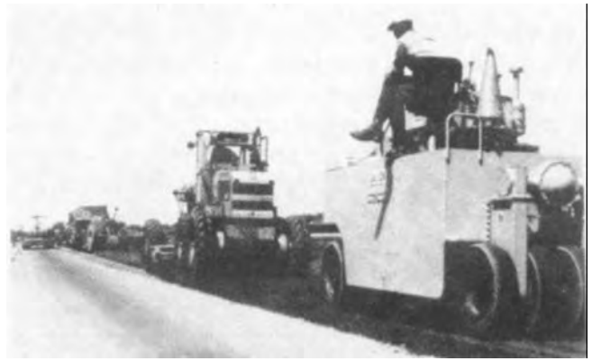
Figure 4-52. Spreading and compacting train.
