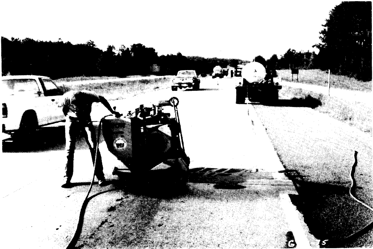
Figure 4-1. Concrete Saw Refacing Joint.
