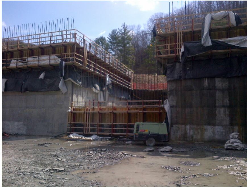
Monolith construction of the right training wall.
