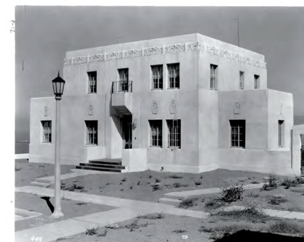
View of Building 11 looking north, c. 1934 . Note the original steel windows and the unpainted terra cotta features. (Courtesy of SFVAMC)
