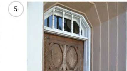
Decorative wood doors, transom, stepped concrete arches at door surround
