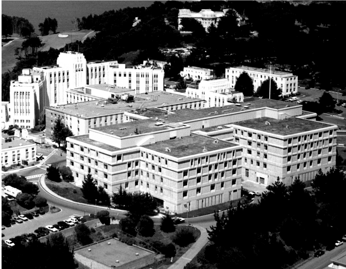
Figure 72. View of Building 203, facing northeast, ca. 1989 (courtesy of SFVAMC).
