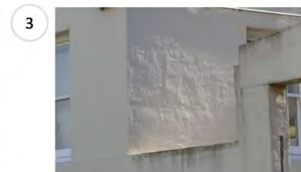
Painted stucco on concrete exterior walls
