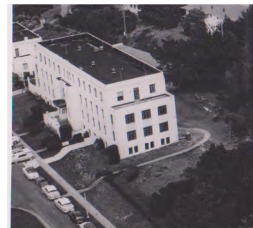
View of Building 8 looking north, c. 1950 . Note the original steel windows, unpainted terra cotta spandrels, and lack of 3rd floor additions on each stepped side wing. (Courtesy of SFVAMC)
