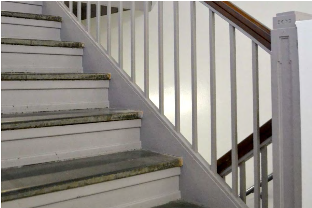
Figure 52. Stairway in Building 1 showing original slate stair treads (photo by HHM, 2014).
