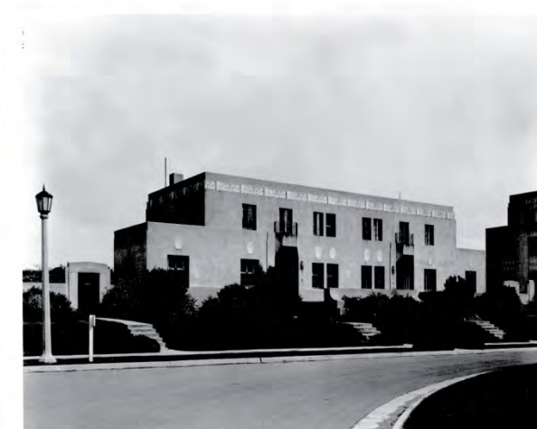
View of Building 9 looking east, c. 1934. Note the original steel windows and the unpainted terra cotta spandrels. (Courtesy of SFVAMC)
