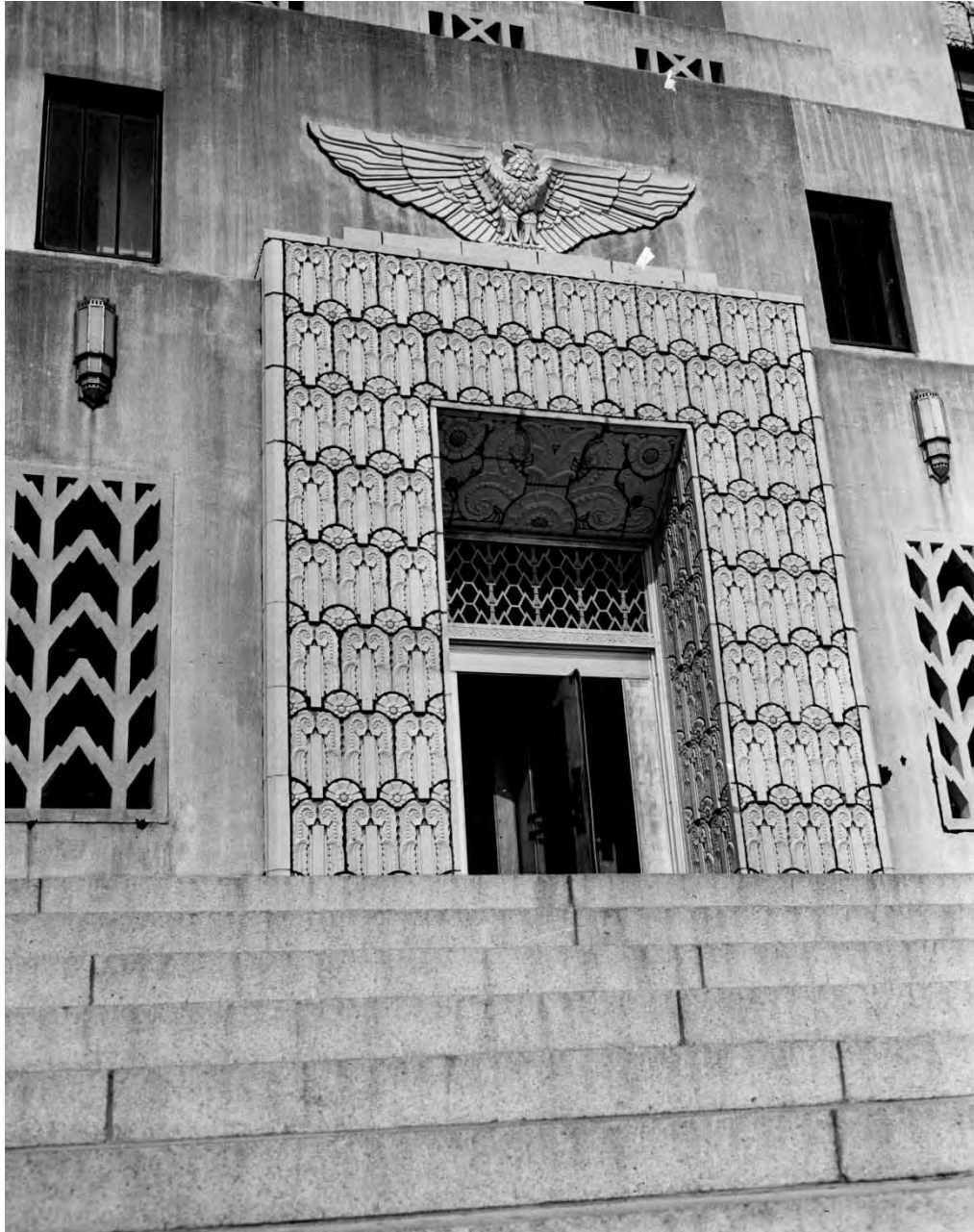
Figure 48. Photograph of the original entrance of Building 2 in 1939, showing the steel revolving door and decorative steel grate at the transom (courtesy of SFVAMC).
