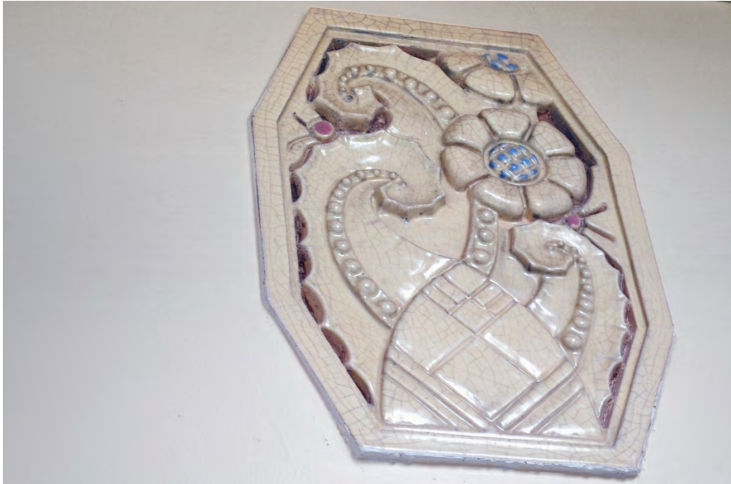
Figure 40. Detail of original unpainted ornamental terra-cotta panel located in Building 11, (photo by HHM, 2014).
