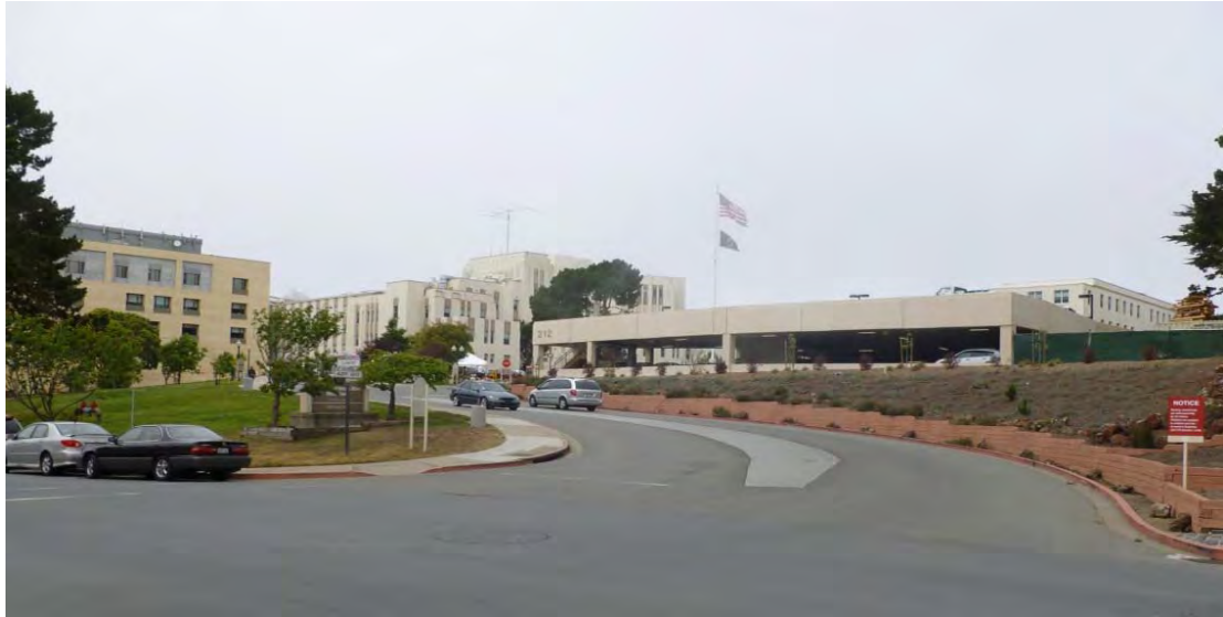
Figure 15. View of campus from Clement Street, facing northwest (photo by HHM, 2014).
