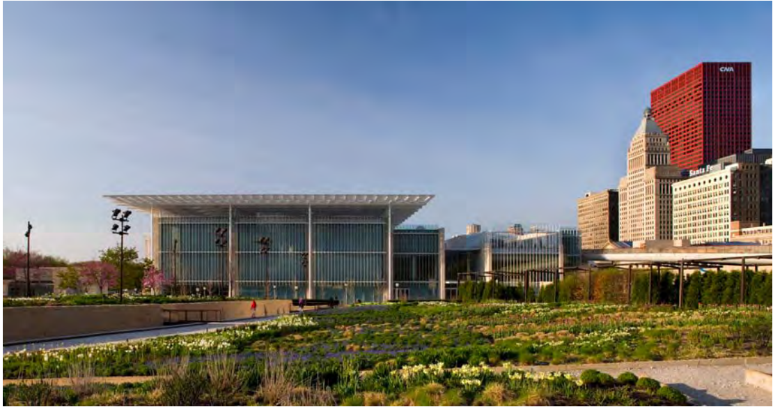
Figure 37. Although the exterior walls of the new building are primarily glass, the color palette complements the materials of the surrounding historic buildings. Modern Wing at the Chicago Art Institute, designed by the Renzo Piano Building Workshop, Chicago, Illinois, 2009, http://www.archdaily.com/24652/the-modern-wing-renzo-piano/262826382_t-m-w-1/ (accessed August 24, 2014).
