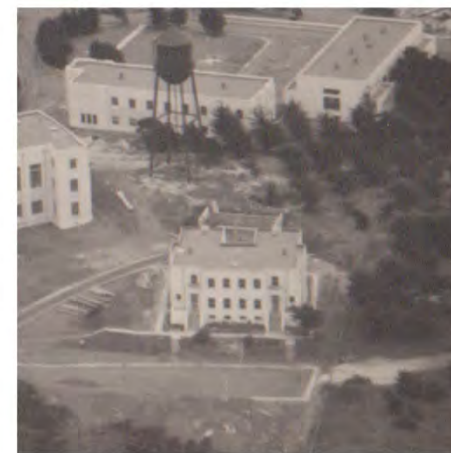
View of Building 18 looking south, c. 1934. (Courtesy of SFVAMC)
