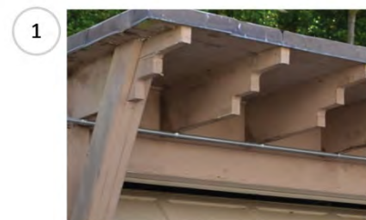
Decorative wood brackets
