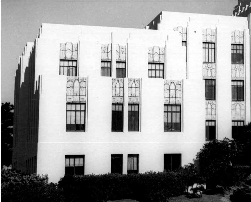
Figure 41. South wing of Building 1 showing original steel frame casement windows, facing west, ca. 1950 (courtesy of SFVAMC).
