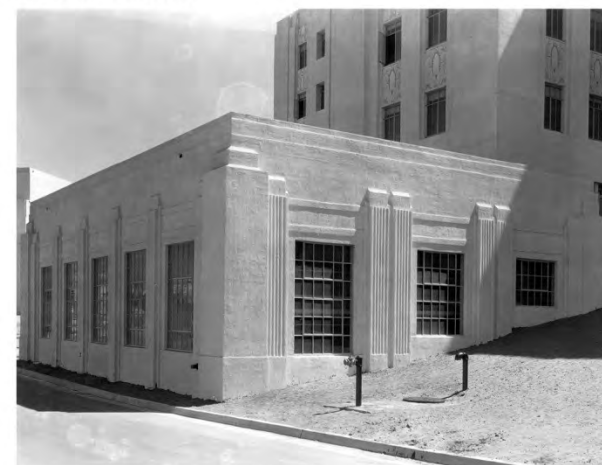
View of Building 3, c. 1934 . Note the original steel windows and larger window openings. (Courtesy of SFVAMC)
