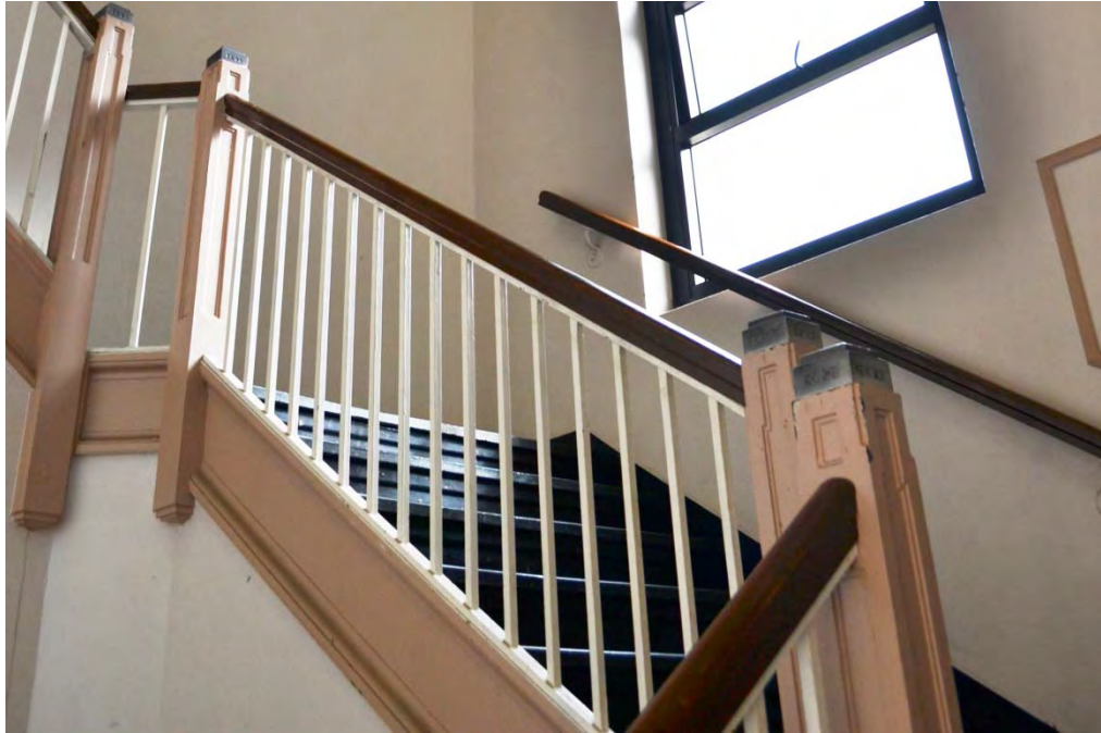
Figure 51. Stairway in Building 7 (photo by HHM, 2014).
