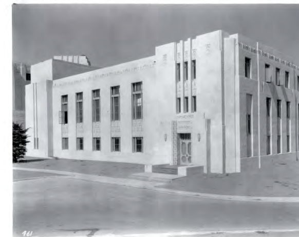
View of Building 7 looking northwest, c. 1934 . Note the original steel windows and doors and the unpainted terra cotta spandrels. (Courtesy of SFVAMC)
