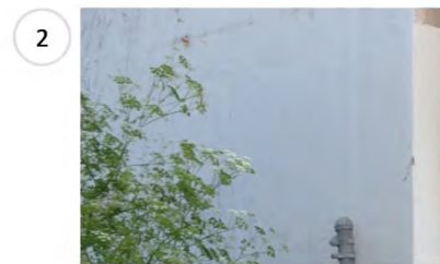
Painted stucco on concrete exterior walls
