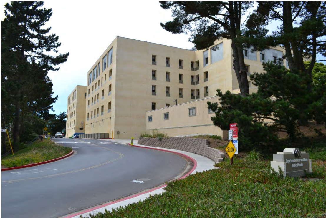
Figure 17. View of campus from Clement Street, facing northwest (photo by HHM, 2014).
