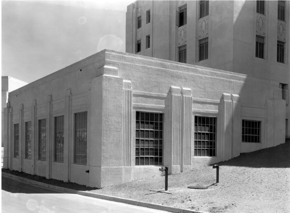
Figure 42. Building 3 showing original steel frame windows, ca. 1934 (courtesy of SFVAMC).
