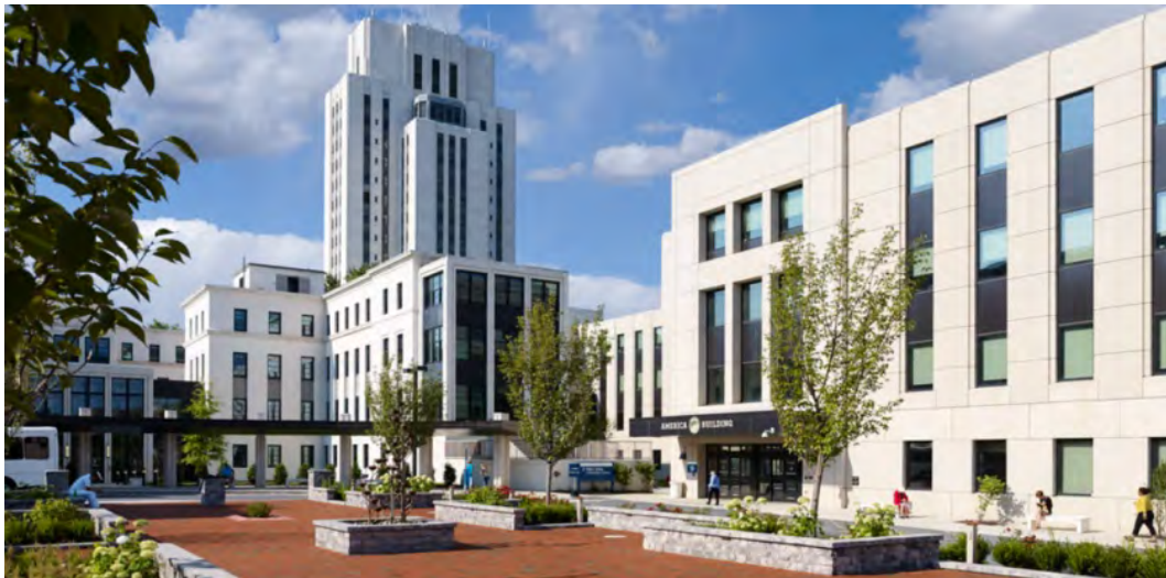
Figure 36. Note how the color, massing, and verticality of the fenestration pattern of the new building on the right all reflect the design of the original historic buildings at the center and yet do not detract from them. National Naval Medical Center at the Walter Reed Military Medical Center in Bethesda, Maryland, designed by HOK, 2012, http://www.hok.com/design/type/healthcare/walter-reed-national-military-medical-center/ (accessed August 24, 2014).
