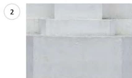
Painted stucco on concrete exterior walls
