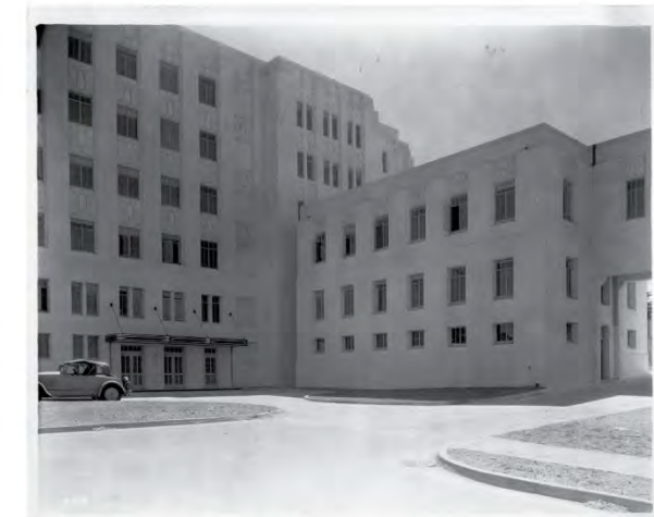
View of Building 4, c. 1934 . Note the original steel casement windows and the unpainted terra cotta spandrels. (Courtesy of SFVAMC)
