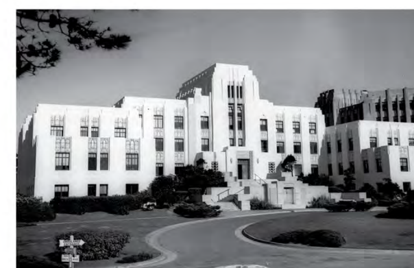
View of Building 1 and landscaped forecourt looking west, c. 1950 . Note the original steel windows and doors and the unpainted terra cotta spandrels. (Courtesy of SFVAMC)
