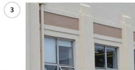
Fluted profile on engaged pilasters between windows
