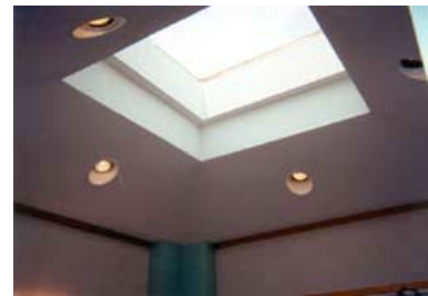
Fig. 15 Skylights in the Helmsman with ample daylight and electric lights turned on, emphasizing the need for controls.
