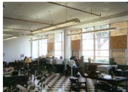
Fig. 17 Building 241 is being considered as a demolition site, but provided the potential as a tremendous renovation opportunity, especially responding to energy and daylighting.
