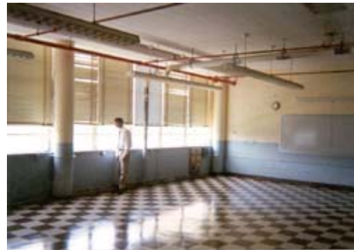
Fig. 11 Building 241 has excellent opportunities for energy efficiency with its ideal orientation and apperatures.
