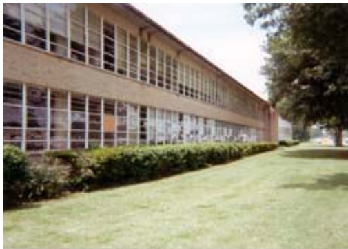
Fig. 12 Building 241 interior provides great daylighting and sun control opportunities with high ceilings and north and south windows.
